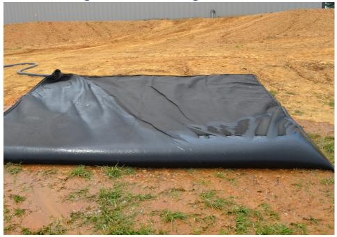
PacTec's SludgePac dewatering bag is the ideal solution for capturing solids from pumping operations. They easily contain silt, soil, debris and sediment while allowing water to safely return to the ground or storm drains.
